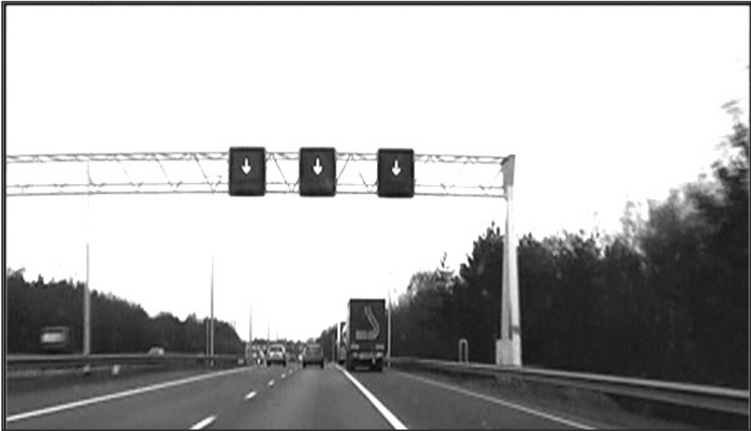
Figure 1: Shoulder Travel Lane with Overhead Lane Controls in the Netherlands
